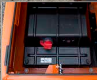
Battery cut-off switch
